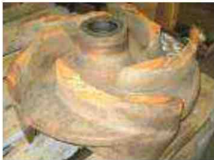
Worn out pump impeller before repair
